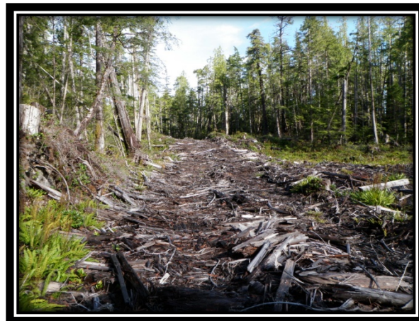
Figure 15: Permanent access wood corduroy road with no fines or sedimentation from harvest related impacts.
